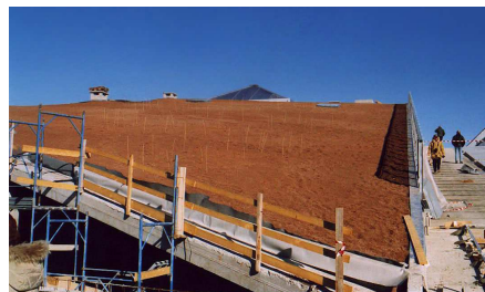
After the substrate layer was applied.
