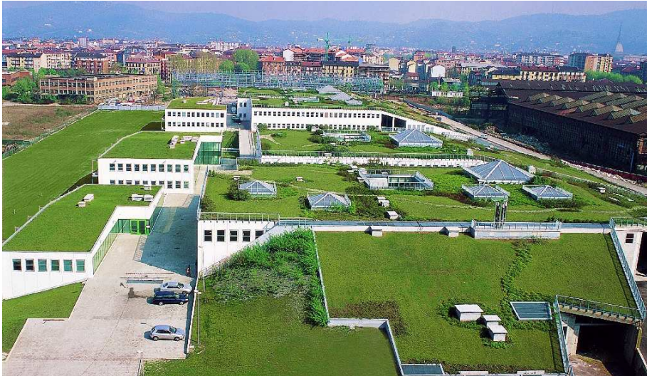
The flat and pitched green roofs of the Environment Park.
